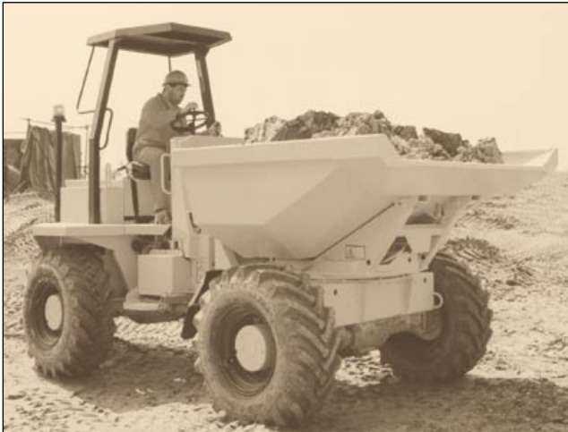
Figure 7 Site dumper with ROPS
